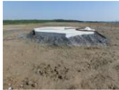
Concrete foundation on a landfill in Chubu district (7m in diameter, 1m thick)
