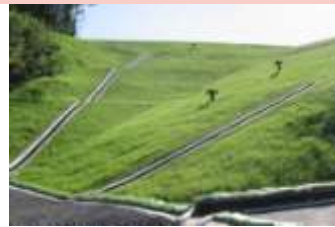
Measured site of illegal dumping
