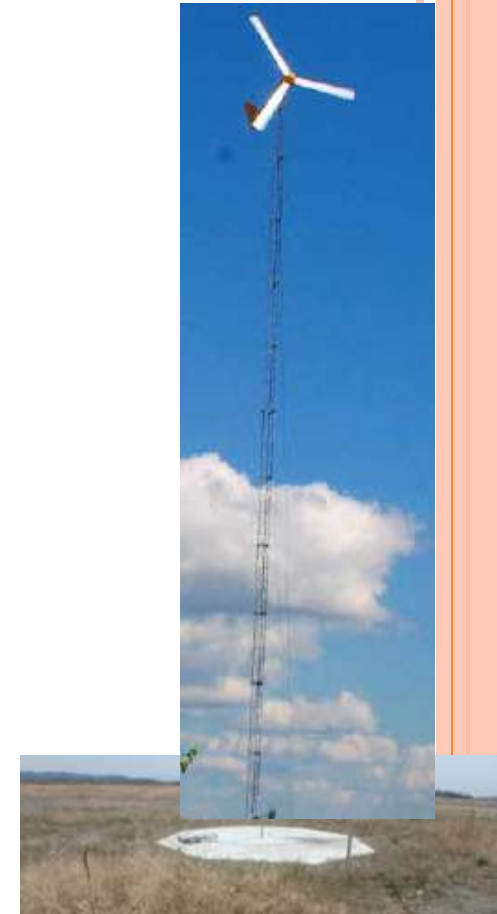
Concrete foundation on a landfill in Chubu district (7m in diameter, 1m thick)
