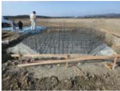
Concrete foundation on a landfill in Chubu district (7m in diameter, 1m thick)
