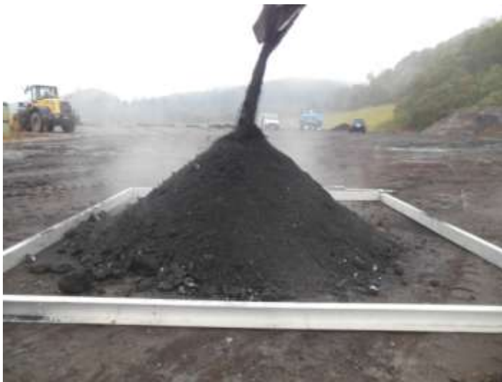
Controlled type landfill in Tohoku
