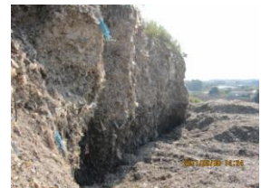
Photograph 1. Upright solid waste wall (Kanto-1 site, after surface collapse)
